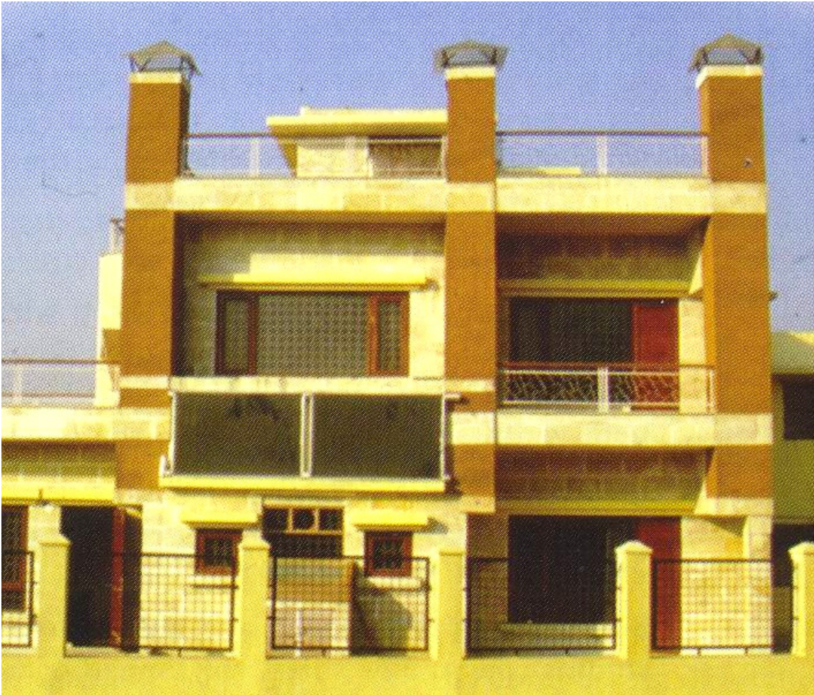
Fig. 6.3 Solar hot water systems in Sudha and Atam Kumar's residence in New Delhi [2]
