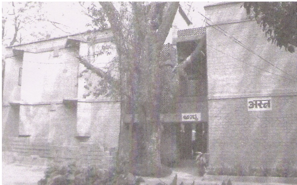
Fig. 7.7 Photograph of ASTRA building, Bangalore
